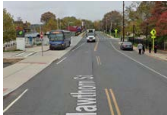
Approach to Sigourney Street CTfastrak Station
