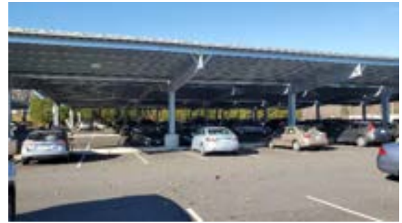
Ground-Level Solar Canopy at UMass Amherst
